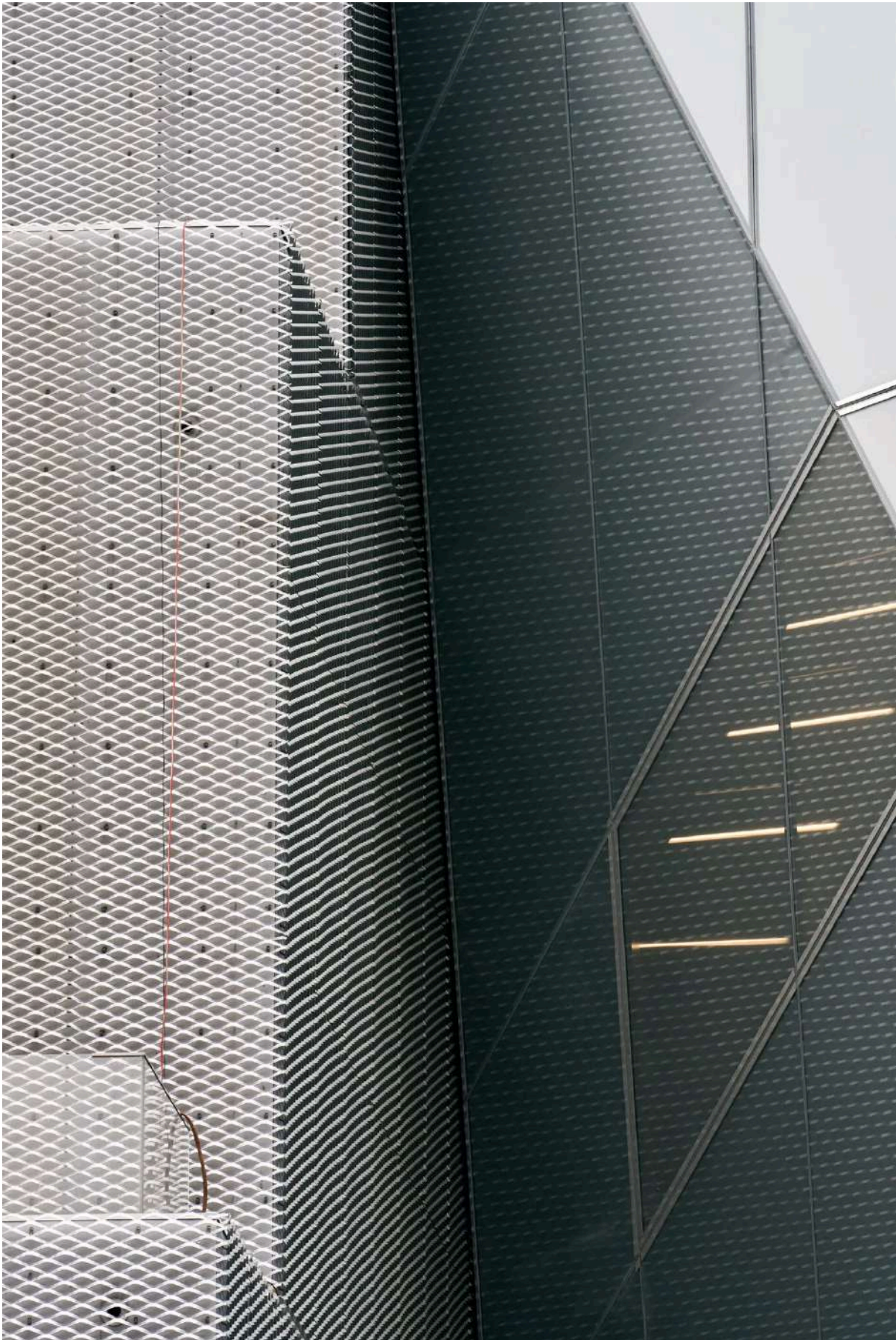
Left, the 2007 New Museum building, designed with stacked, off-axis boxes by the Japanese architecture firm SANAA (Kazuyo Sejima and Ryue Nishizawa). Its aluminum mesh facade now “kisses” the new addition, right, by OMA.
