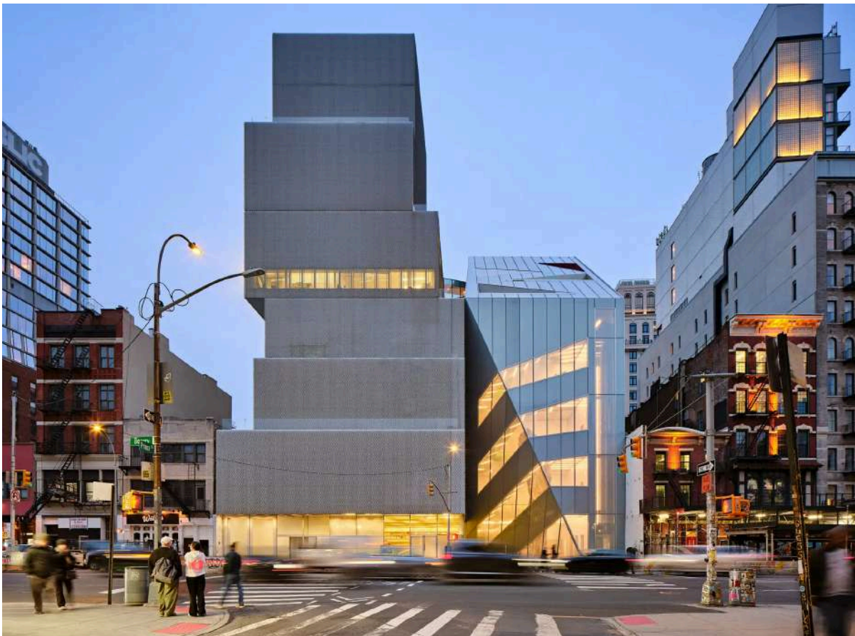
The New Museum, on the Bowery, in 2026, with its stacked boxes at left, designed by SANAA, and the addition at right by the OMA partners Rem Koolhaas and Shohei Shigematsu. via New Museum; Photo by Jason Keen
